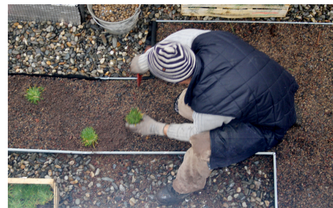
Plantation of micro-clumps on a green roof © Le prieuré
