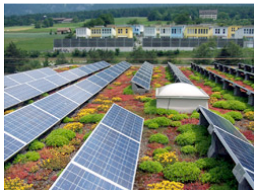
Green roof and photovoltaic combination © 2018, International Green Roof Association
