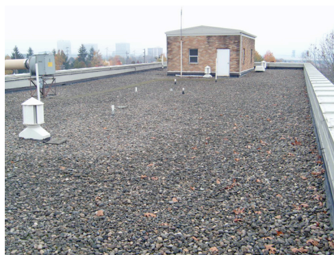
Gravel roof © Anderson Roofing
